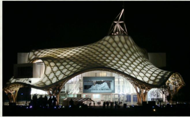
Centre Pompidou Metz(France) Architect:Shigeru Ban Architects Europe & Jean de Gastines GC:Demathieu & Bard
