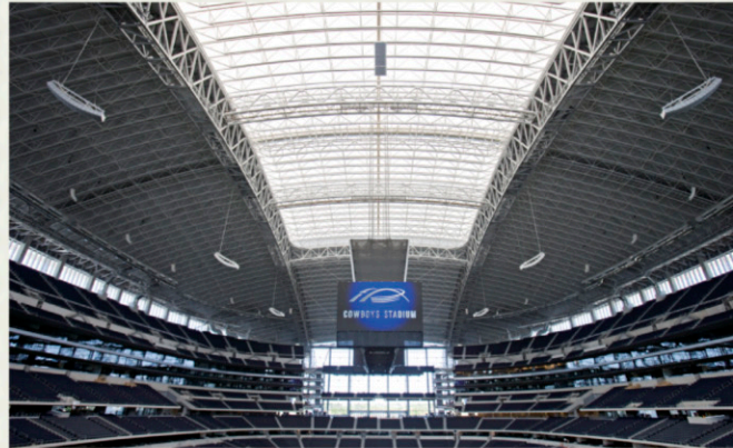
Dallas Cowboys Stadium(USA) Architect:HKS, Inc. GC:Manhattan Construction
